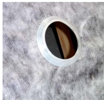
Seal ring installed.
