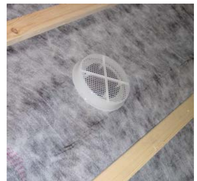
The mesh cover in place.
